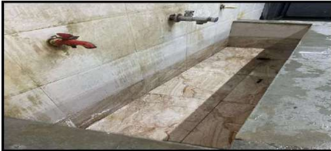
TIFFIN-PLATE CLEANING WASHING AREA
