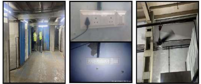
FACILITY FOR WORKERS (FAN, LIGHTS, CHARGING POINTS)
